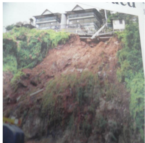
Pic 2: landslide damage to natural environment and Residential house along Ports Road in Town Area
