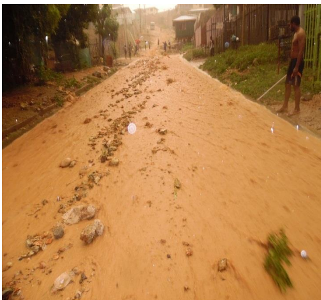
Pic 1: Flood and soil erosion of Hilltops developments during Heavy downpour at Ranbo Estate
